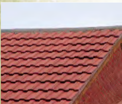
No chimney or flue
